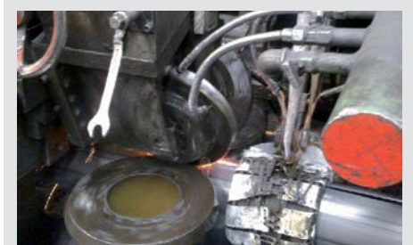
Temperature monitoring of pipe rims shortly before welding
