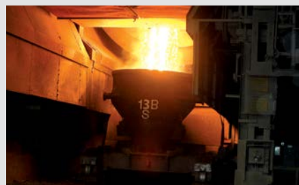
Monitoring of the refractory lining of a slag ladle car while pulling out of the factory
