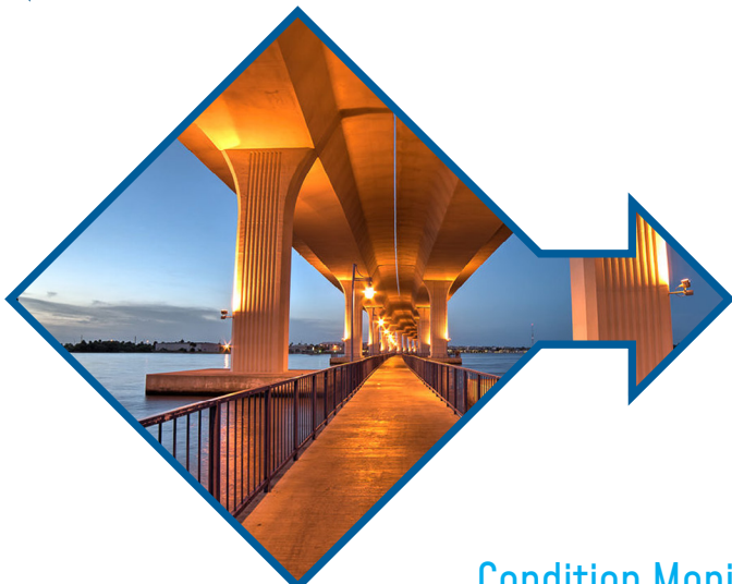
Structural Health Monitoring
