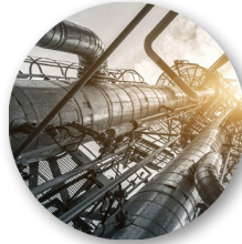
AIR-CONDITIONING SYSTEM (HVAC)
